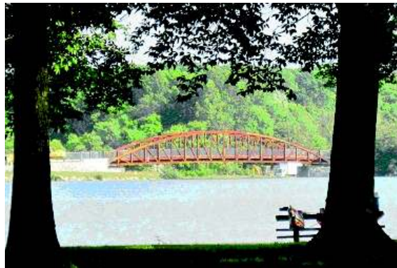
Deer Creek Bridge Lexington Township
