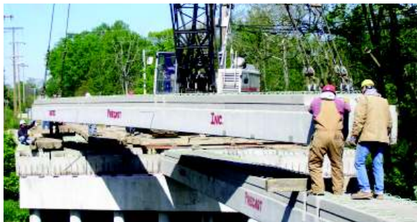
Wooster Street Bridge Village of Navarre
