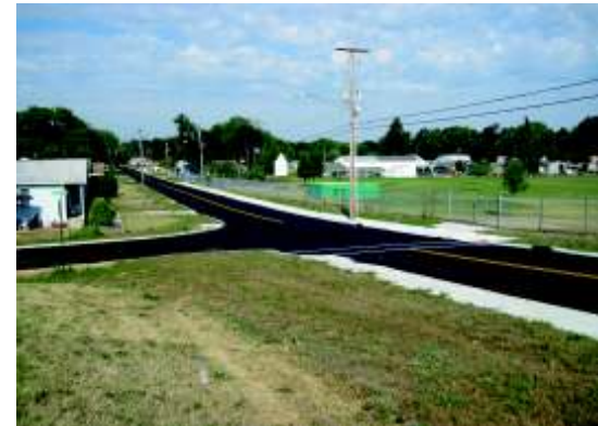
Plain Twp. - 25th St. Storm Sewer
