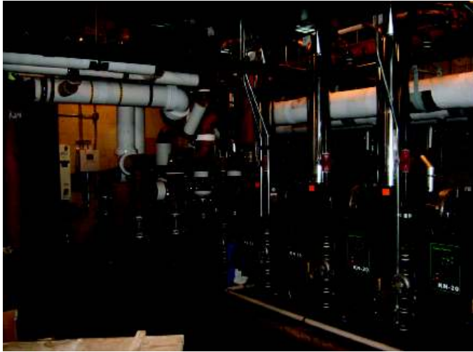
New Boilers Stark County Jail
